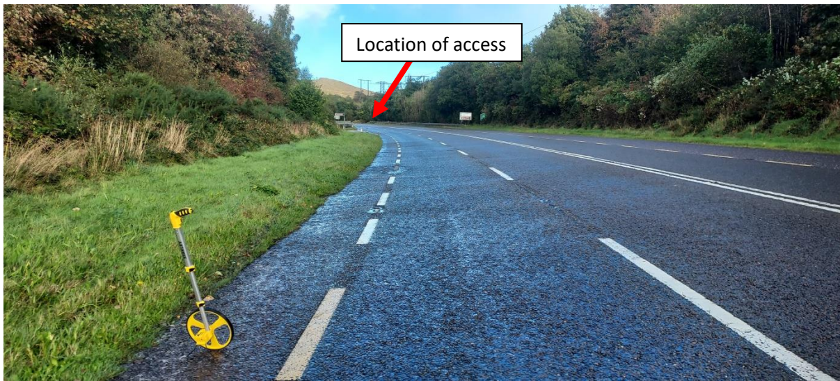
Plate FI5 Looking northeast towards existing Kilgarvan Wind Farm access junction on N22 – forward visibility from point 215m from access junction available
