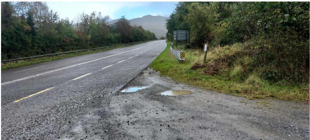
Plate FI2 Taken from existing Kilgarvan Wind Farm access junction on N22 – looking northeast – visibility of 215m along nearside of hardshoulder available from 3m setback
