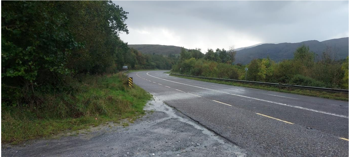
Plate FI1 Taken from existing Kilgarvan Wind Farm access junction on N22 – looking south west – visibility of 215m along nearside of hardshoulder available from 3m setback
